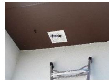
WH Ventilation Runtime
