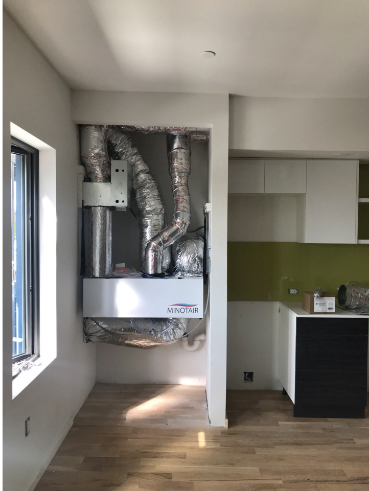
HVAC Closet merged with Kitchen cabinetry
