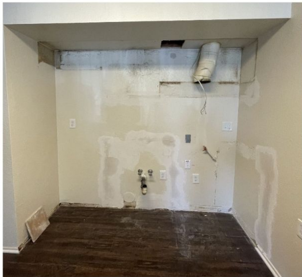
WEDNESDAY Site Preparation
