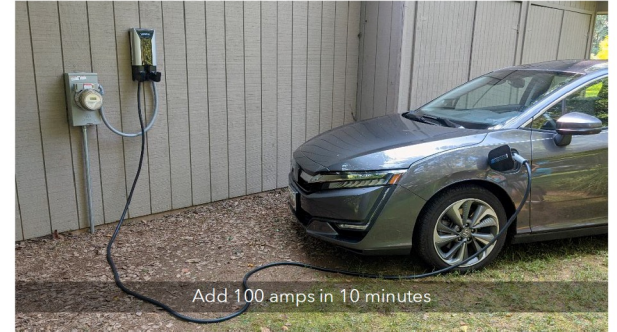
Plug-in adapter uses meter socket instead of the service panel
